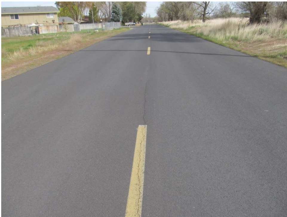
Photo 2: Faler Road (Mt. Hood Avenue to Mt. Adams Avenue) - Condition Rating "Good"
