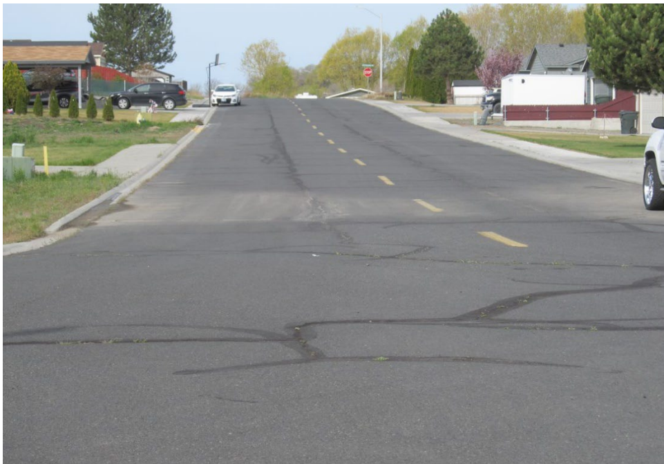
Photo 4: Pheasant Court (Looking West toward River Ridge Drive) - Condition Rating "Fair"
